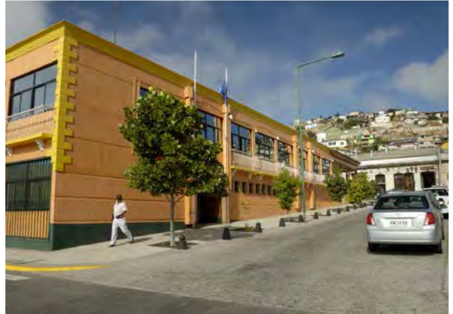
Edificio Aduana, Plaza V Mackenna (Puerto) / Customs Office Building, Vicuña Mackenna Square (Port)
